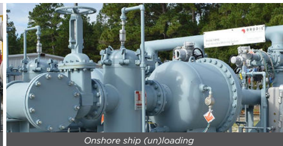
Onshore ship (un)loading
