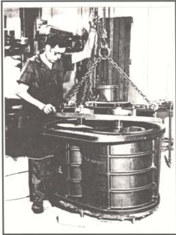
Figure 4.10 Position and lower rear end plate in place
