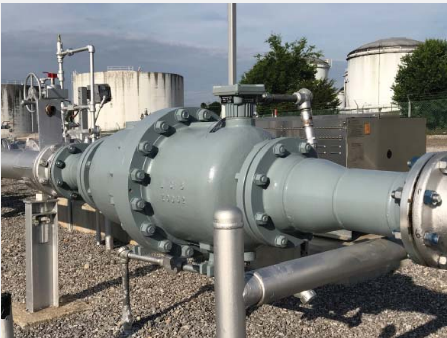
Brodie's 8" BiRotor Plus PD meter in place of a helical turbine meter.
